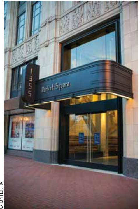
The entrance to the new lobby near Ninth Street
