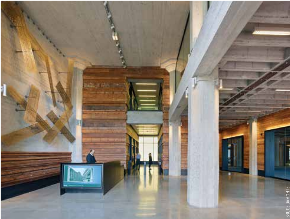
The new Ninth Street lobby, converted from a former parking entrance, features repurposed Douglas fir that was found in a wooden structure on the roof of the building.
