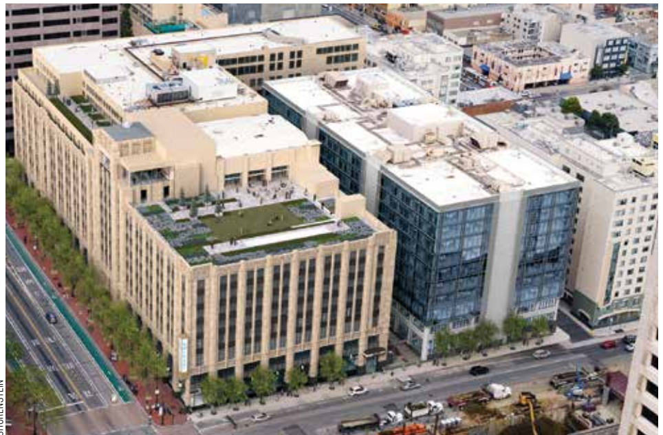
The buildings before (top) and after renovation, highlighting the new roof deck and the new glass curtain wall for the 1 Tenth building.
